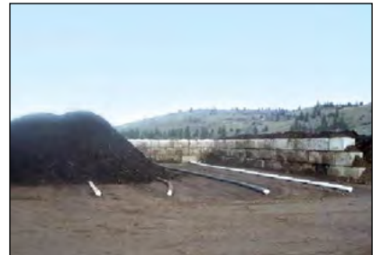
Photo 5-13: Typical ASP system with aboveground piping; block walls separate batches to better utilize available space © CH2M HILL
