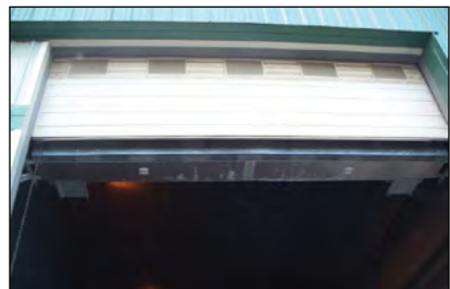
Photo 10-5: Air curtain installed overtop an overhead door © CH2M HILL
