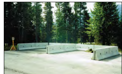
Photo 5-6: Small bunker composting system © Scott Gamble
