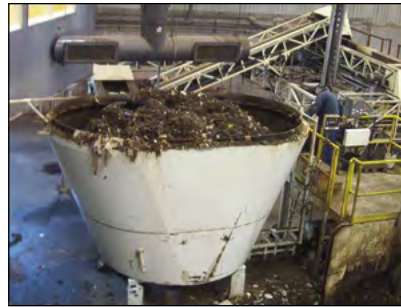
Photo 11-3: Vertical auger mixing unit © Scott Gamble
