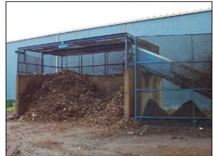
Photo 15-4: Enclosures around screener discharge conveyors help to contain litter © Scott Gamble
