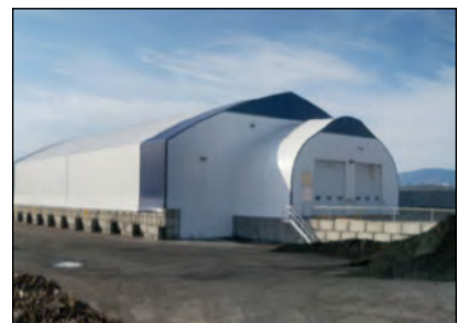
Photo 10-2: Fabric-style receiving building © CH2M HILL
