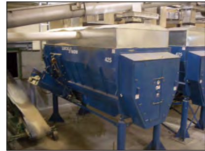
Photo 11-5: Horizontal auger mixer © CH2M HILL
