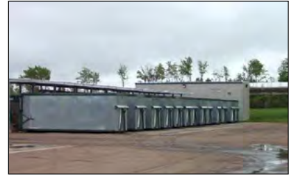
Photo 5-21: Composting system that uses multiple static containers © CH2M HILL
