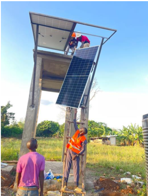
Installation of solar panel
