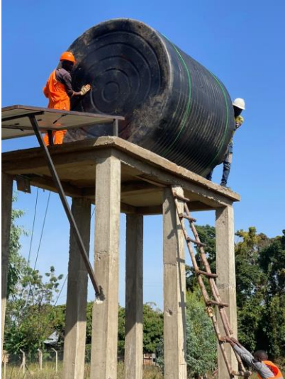
Engineers install in water tank
