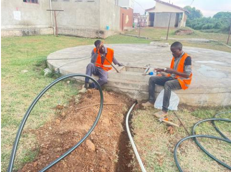
Connecting the pipe system
