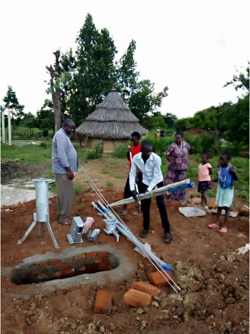
Priming down hole cylinder
