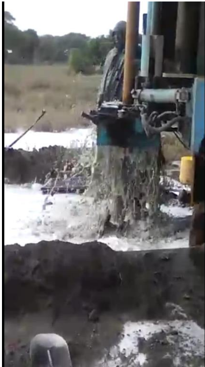
Drilling rig hitting water
