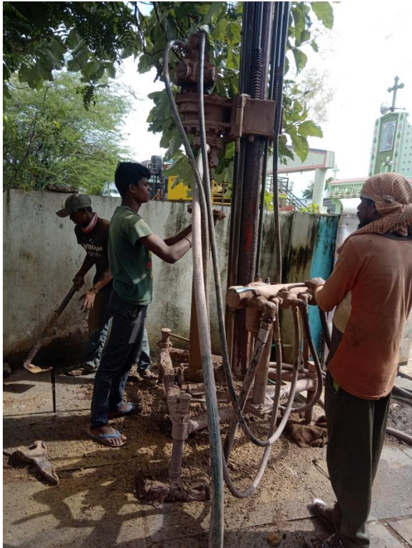
Drilling a bore hole
