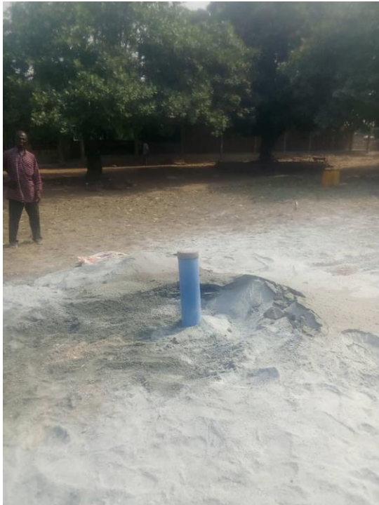
Drilling complete and electrical work in prep for pump
