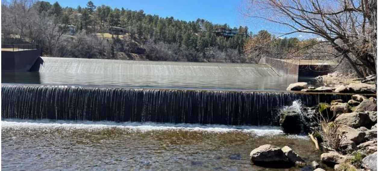
Figure 13: A series of three dams are located at the outfall of Canyon Lake.
