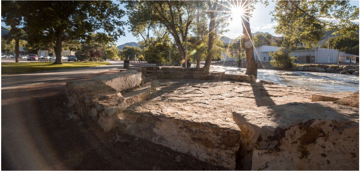
Figure 27: Riverside Patio at the Calibre-designed Canon City Whitewater Park
