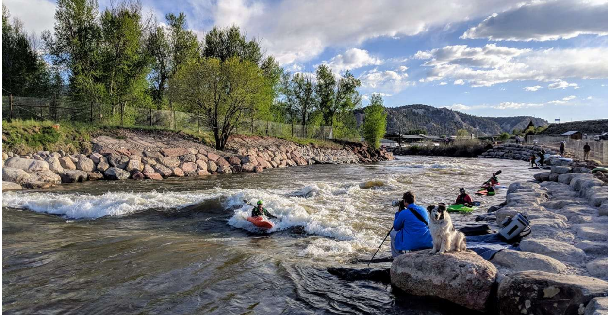
Figure 23: A kayaker surfing in a designed wave in Eagle, CO at high flows.
