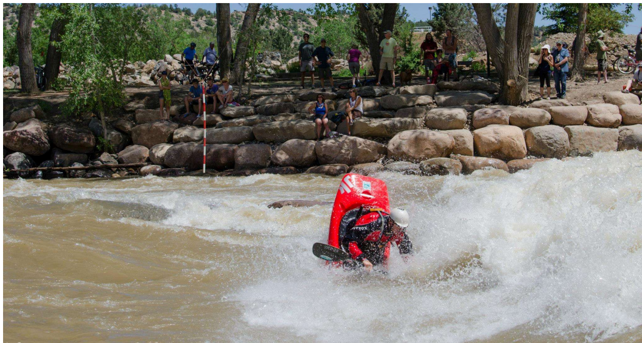
Figure 25: Terraced banks provide flood armoring, streamside seating, and river access. Photo of Calibre-designed Durango Whitewater Park.
