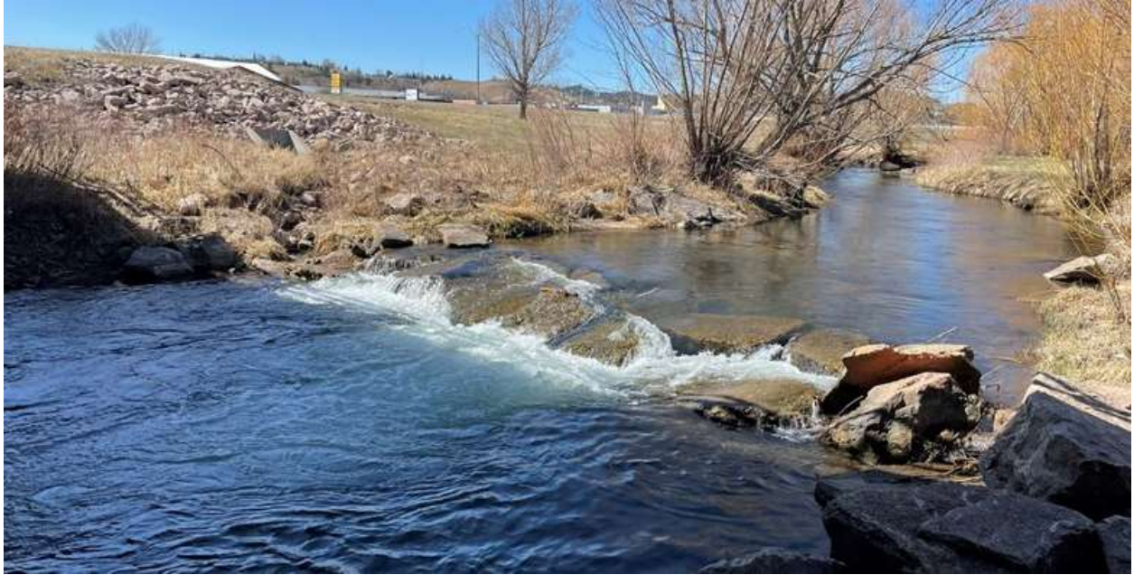
Figure 19: There are numerous drop structures along the reach, some of which are fun to surf or kayak on at varying levels. However, some of these can also be dangerous in their existing condition depending on water levels.
