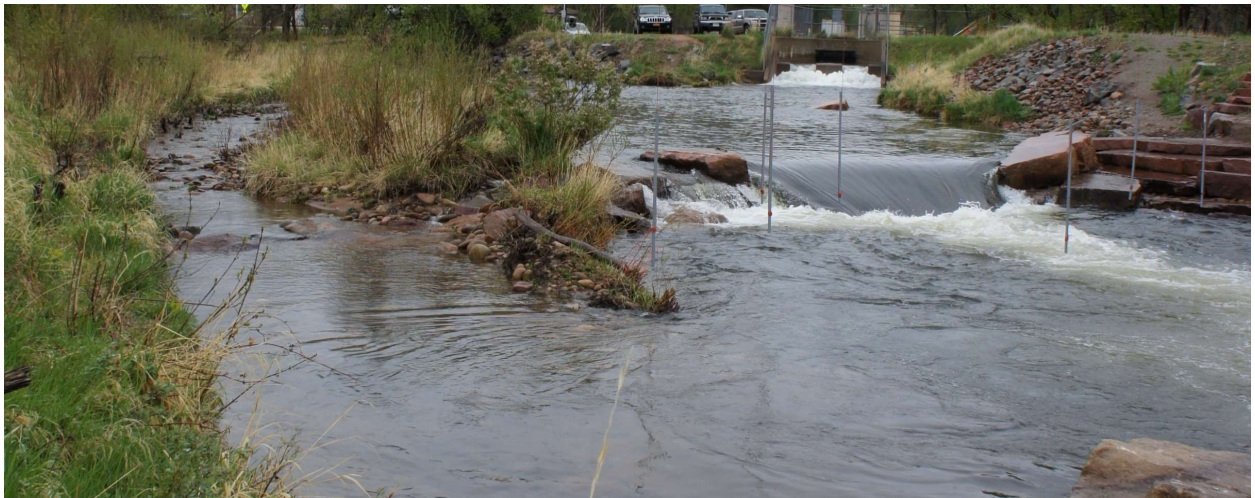
Figure 32: The Calibre-designed whitewater Park in Lyons, CO illustrates a dual channel design (facing upstream). The channel carrying the primary flow has a wave feature (with slalom gates hung), and the secondary flow channel is a constructed boulder riffle that changes grade gradually. This secondary channel was designed to offer fish passage and improved habitat but demonstrates a similar configuration to the dual channel for a play stream.
