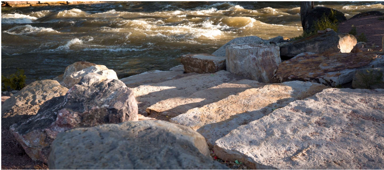
Figure 26: Steps made of slabs of stone offer convenient access and a natural appearance along the bank (Canon City Whitewater Park)
