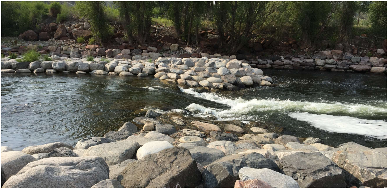
Figure 22: A Wave Structure is constructed of natural rock and grouted into place. The feature pictured is low flow through the structure at the Calibre-designed Eagle Whitewater Park
