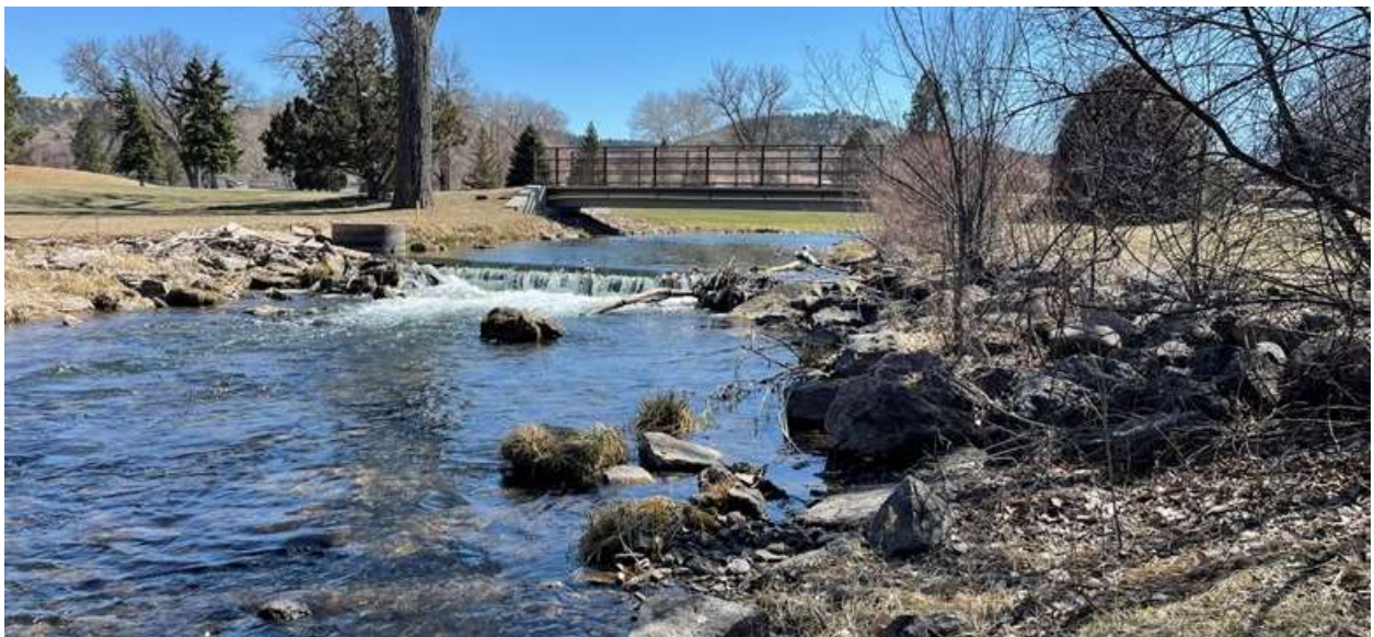
Figure 14: A small dam is located near the Meadow Brook Golf Course, shortly upstream of Jackson Blvd
