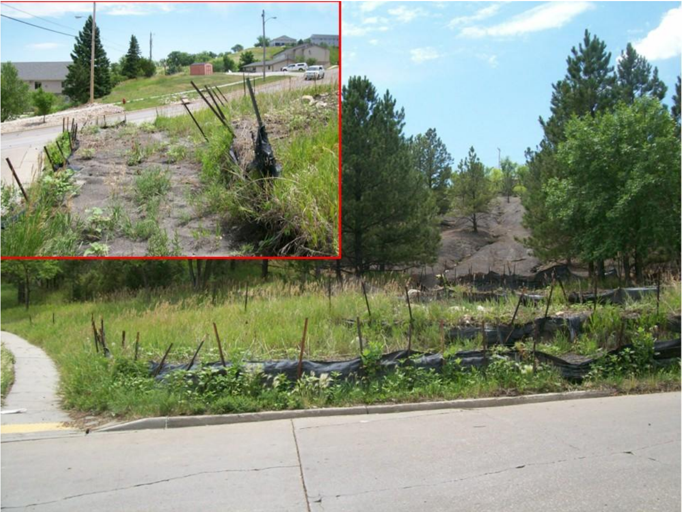
Figure 3. Photos showing dilapidated silt fences. Main photo is looking south and inset photo is looking east.
