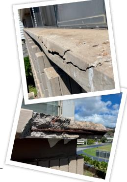
Top: What looks like a small crack or chip in the concrete may not seem serious to the untrained eye, but it can indicate deeper problems beneath the surface.
