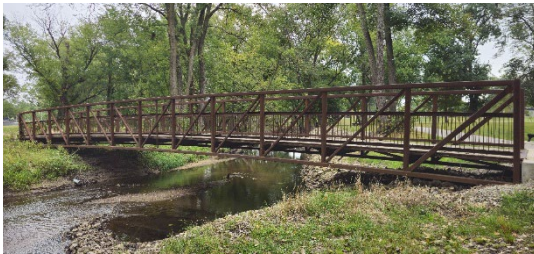
Bridge Traversing Both Parks
