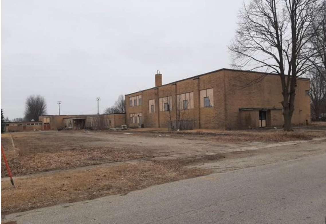
Belmond-Klemme School before the asbestos remove and demolition | Photo Credit: City of Klemme
