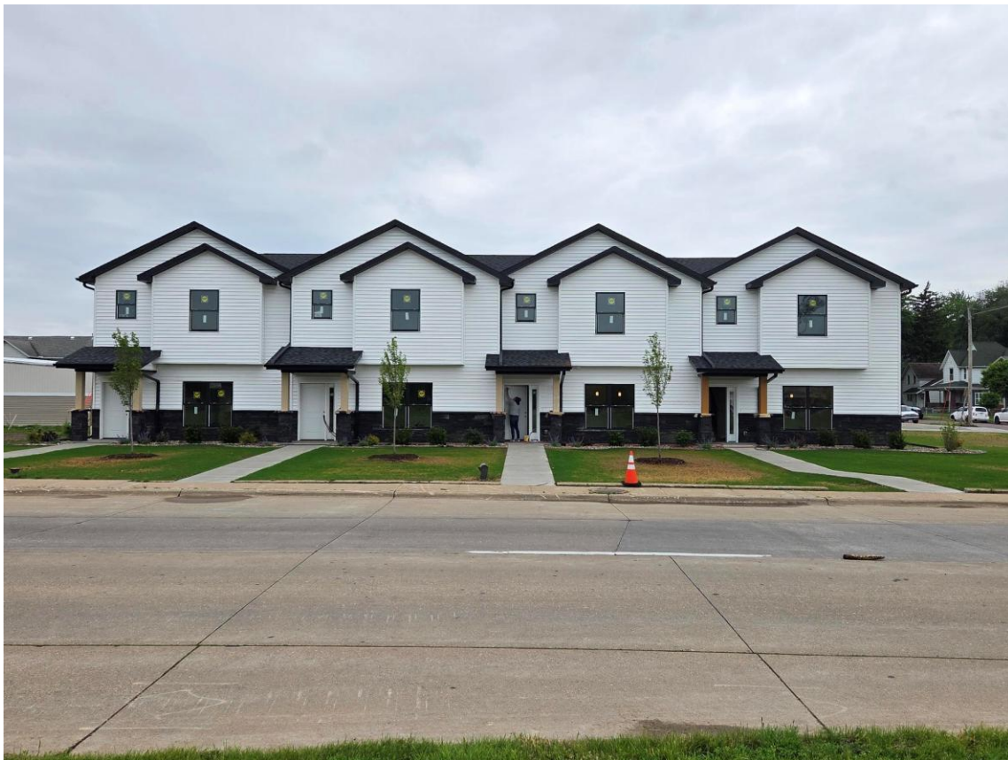
Energy Efficient Townhouses | Photo Credit: East Central Intergovernmental Association
