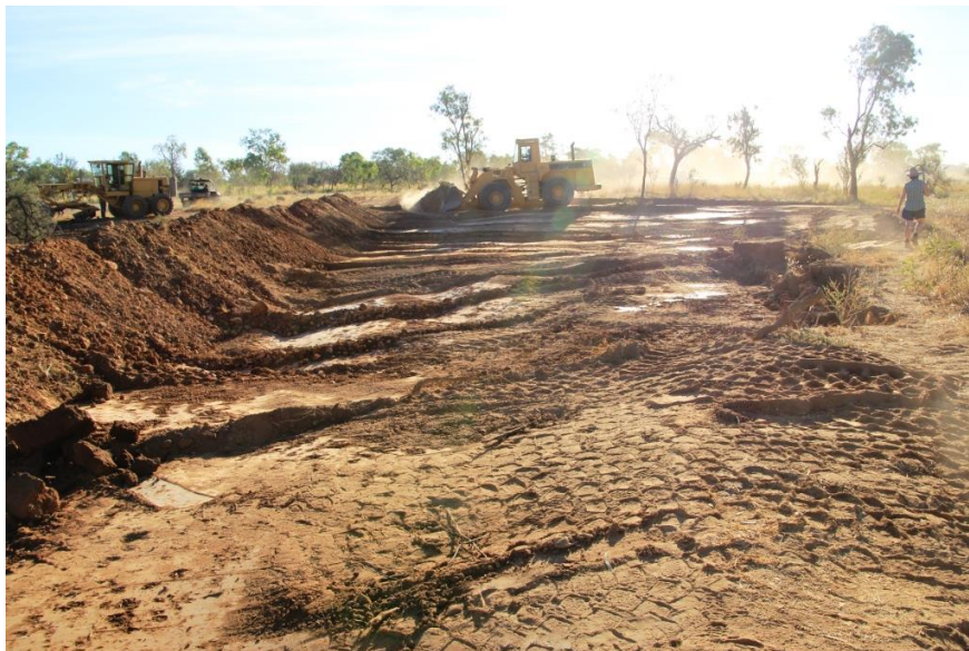
Head of the erosion being levelled, and wall being built
