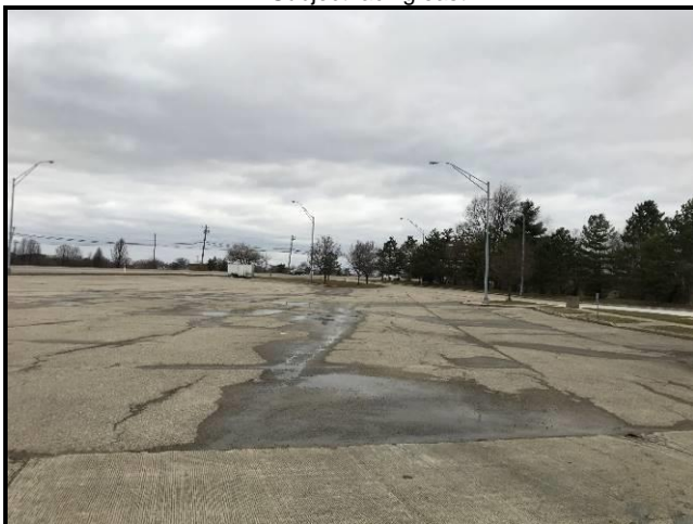
Subject facing northwest
