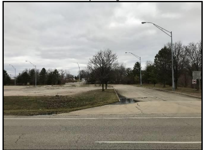
Eastern entrance facing north
