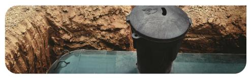
that your underground tank is placed in an area that is not subject to vehicular traffic. Underground tanks should be placed well away (at least 10 feet) from any road, street, driveway, or parking lot, at a safe enough distance that vehicles traveling in these areas will not strike or run over the underground tank dome.
