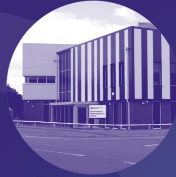
Longbridge Campus Construction & Building Services Centre
