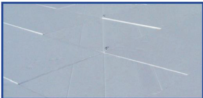
EPS insulation can be cut to shape with a knife or saw to assure a tight fit and eliminate heat loss channels.
