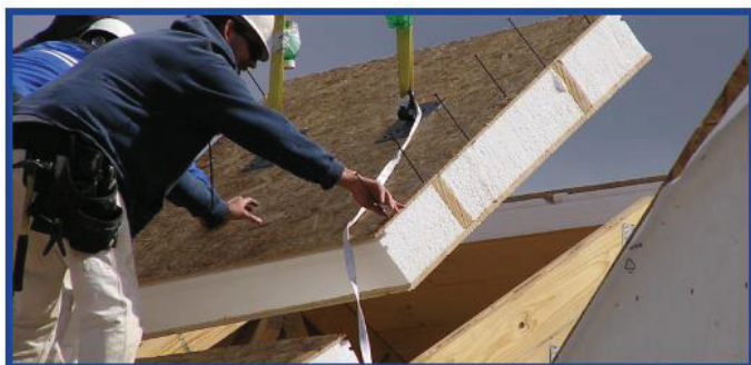
Its light weight allows ease in handling and storage, and in hoisting the material onto the roof.
