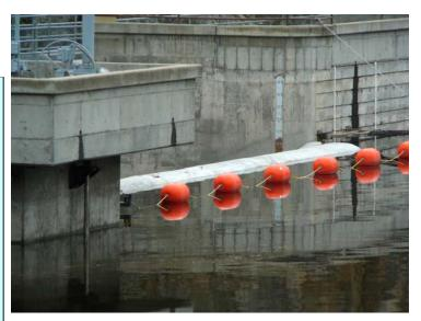
As of Wednesday, May 25, Stagecoach reservoir is almost to the top of the new dam. It has less than a foot of the new 4-foot extension left before the water starts going over the top. Water is being let out through the power plant below at near maximum levels; water blasts out and hits the far side of the Yampa River gorge.
