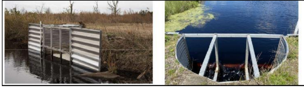
Figure 4. Wetland restoration can be achieved by managing water levels through the use of water level control structures (left) and ditch plugging (right).
