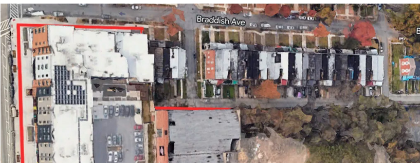
FOCUS AREA 1: Walbrook Mill Apartments
