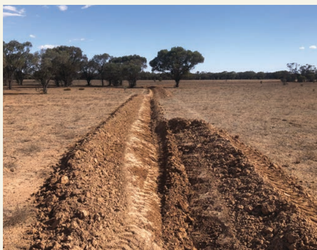
Low profile contour banks were installed in December 2020 including gaps to allow the safe and slower passage of overland water.
