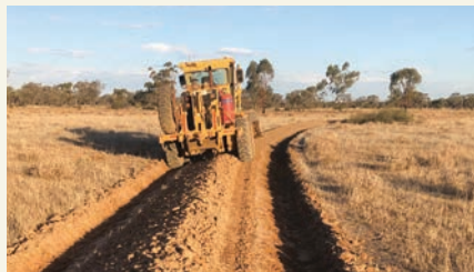
Installing low profile contour banks to slow damaging flood waters.
