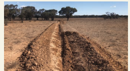
Gaps were left in the low profile contour bank to allow safe and slow passage of overland water.
