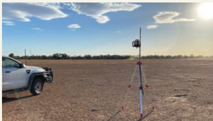
Using laser accuracy to get levels for erosion mitigation works.
