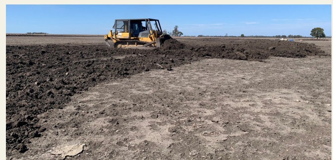
Image 1: Constructing a broad-based contour bank.
