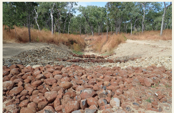
Image 2: Gully rehabilitation works in North Queensland.
