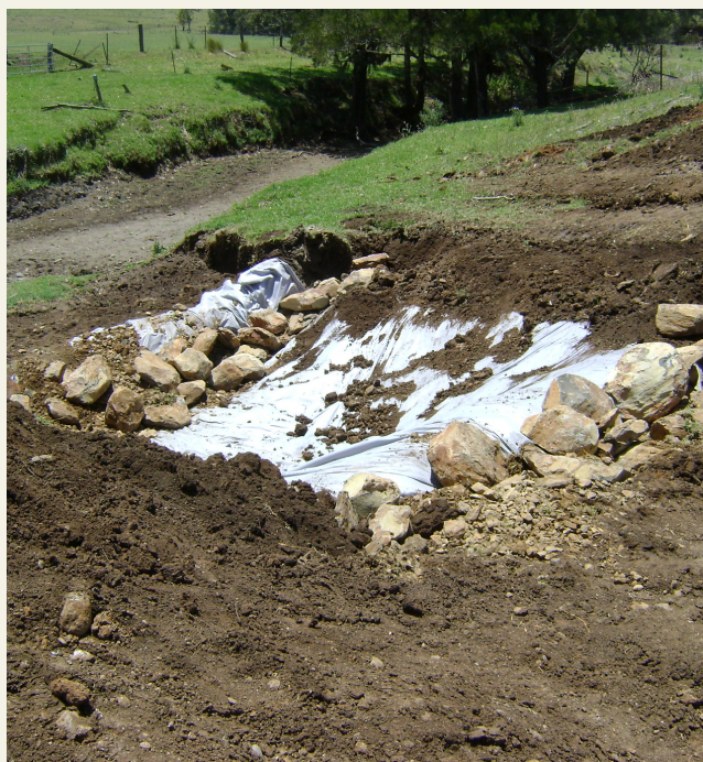
Image 3: Rock chute construction.
