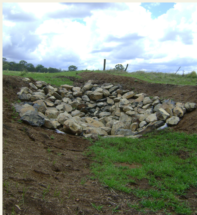
Image 4: Chute for controlling eroding gully head.
