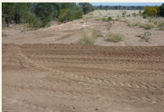
Image 1: Before and after whoa-boy construction. Note erosion to the left of the track in the before photo.
