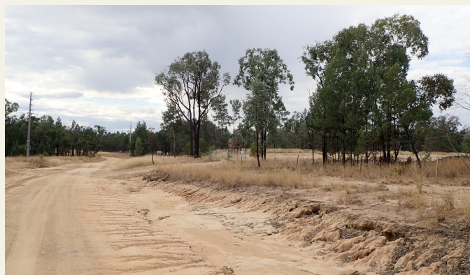
Image 7: Runoff from roads may cause gully erosion.
