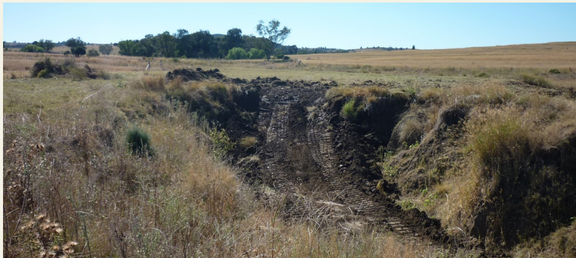
Image 3: Forming an earth ramp to batter the gully head.
