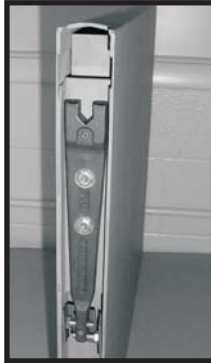
Figure 1a: Centering Bracket in top of door.
