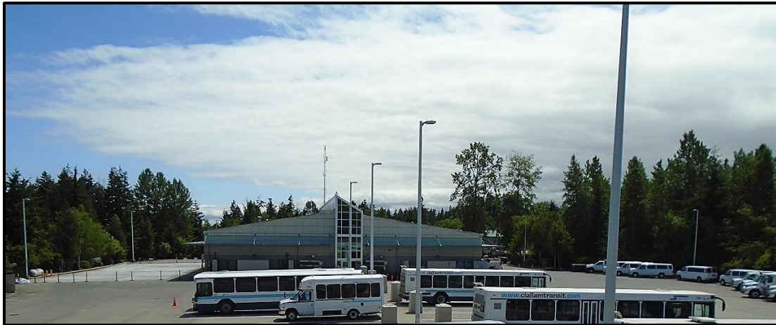
CTS Maintenance Yard and Shop Facility
