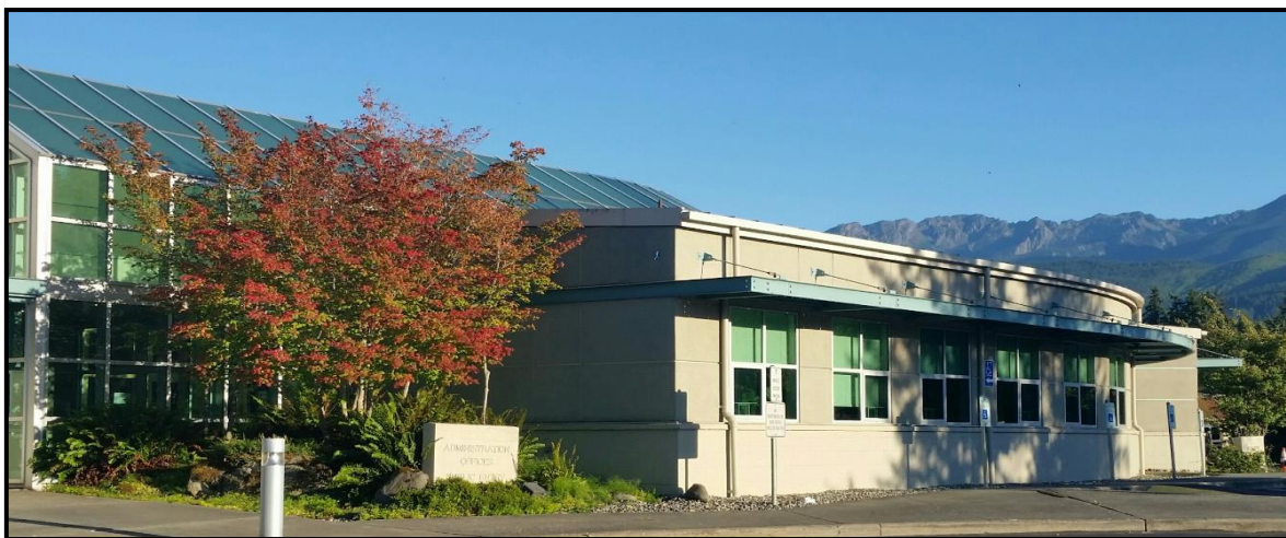
CTS Main Facility – Operations and Administrative Offices
