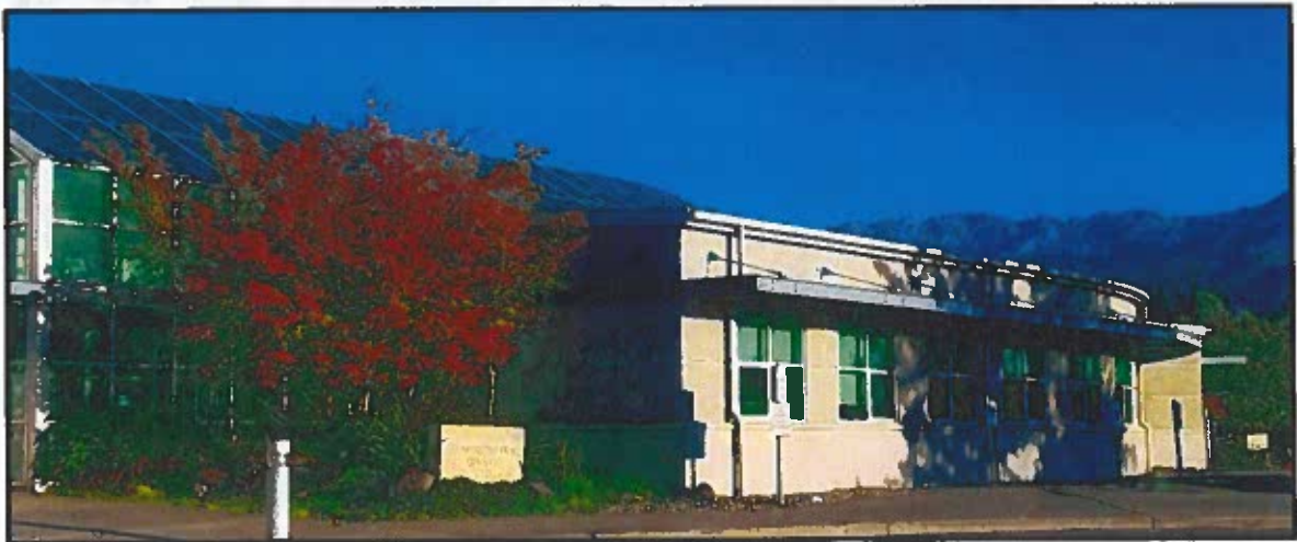
CTS Main Facility – Operations and Administrative Offices
