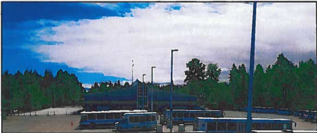
CTS Maintenance Yard and Shop Facility
