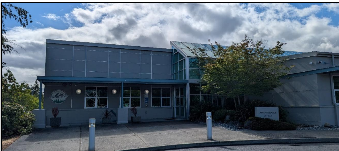
CTS Main Facility – Operations and Administrative Offices
