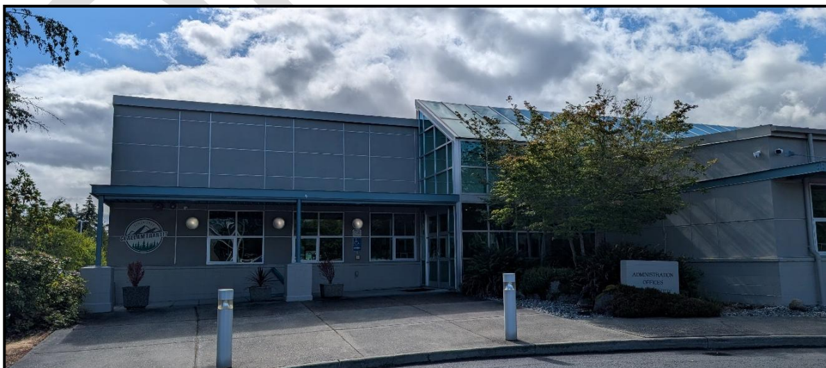
CTS Main Facility – Operations and Administrative Offices
