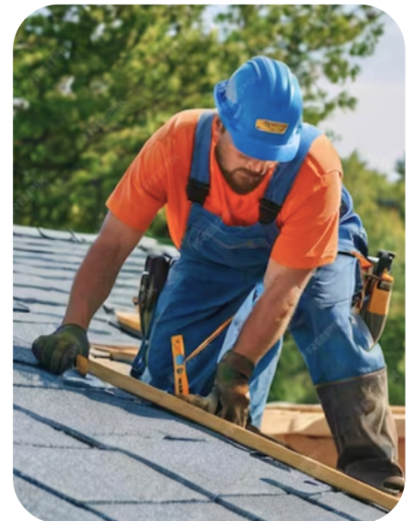
Roof repair technician • Photo: Happy Days Roofing, Lehigh Valley
