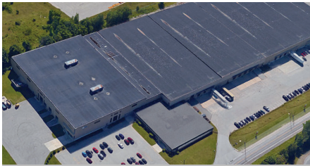
Barrie, ON (CAN) - High Performance Doors
