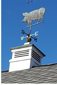
e & After Watson, Repaired 1-
