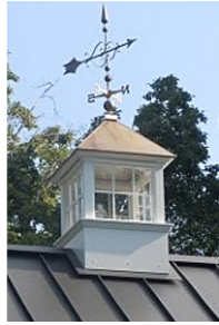
on metal roof with #366-M Lo
