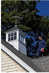
/C (20 year roof, new base & v
