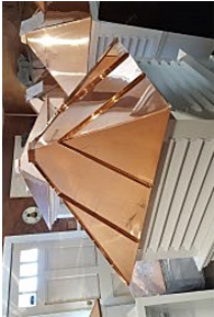
Standing Seam Roof
