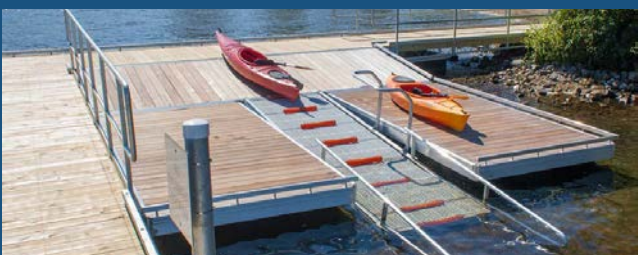
Pathway, bridge and recreational amenities
