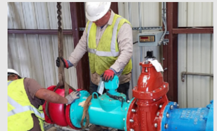
Well Rehabilitation at Tracy Defense Distribution Depot, Tracey, CA, USACE Sacramento
