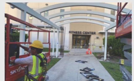
Construct Overhead Protection, SOUTHCOM, Doral, FL
