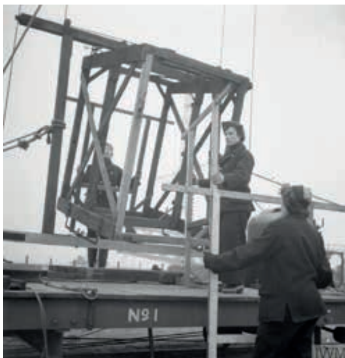
ATS women dismantle Velocity Screens at Shoeburyness
