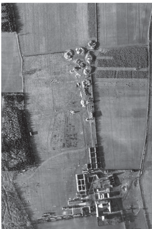
Aerial photo taken in 1945 showing the whole Battery with, to the left, the 4 Gun Emplacements set in a semi circular arc around the oblong Command Post
