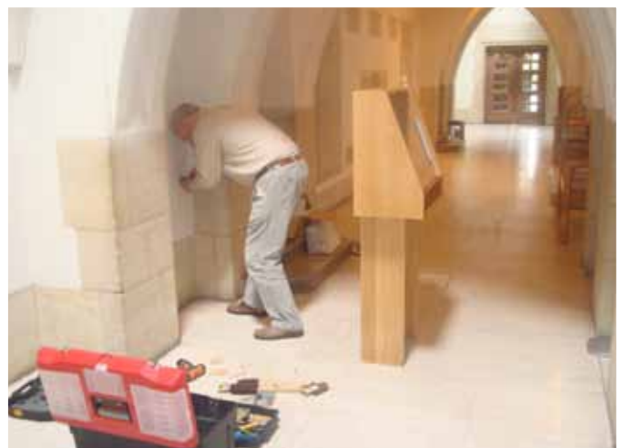
Ron Emmett installing the Memorial Cabinet
