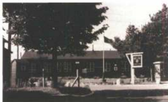
HQ Building WRAC School of Instruction
