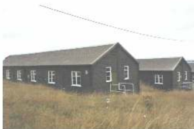
General view of the accommodation
