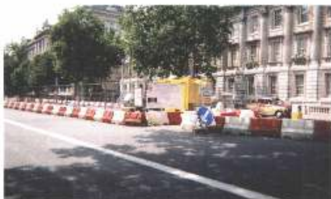
Preparatory Works – June 05
