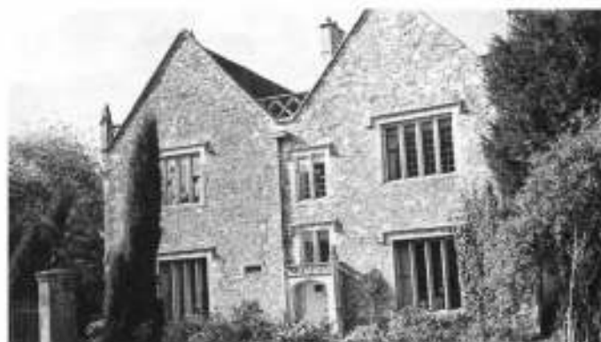
Former WOs and Sgts Mess, now a private house
