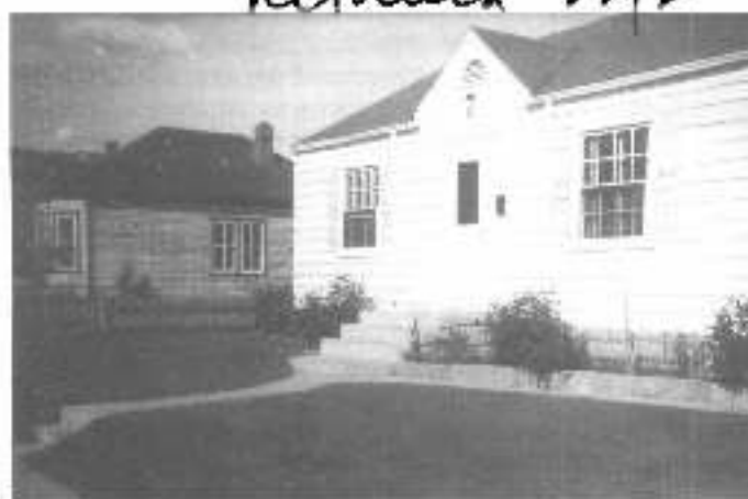
SAME HOUSE AFTER CONVERSION
