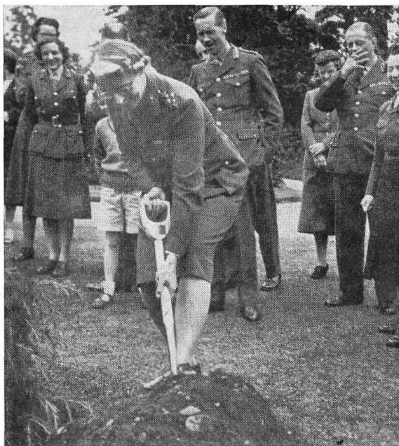
Dame Mary Railton turns the last sod at the W.R.A.C. Staff College
