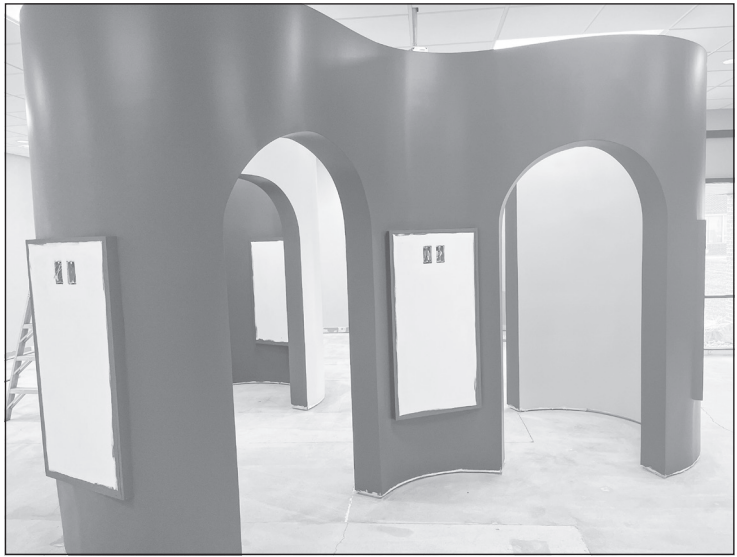
The curved walls of this interactive display nears completion on Tuesday, April 14.
