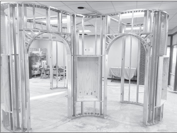
This photo depicts the framing for the curvature of this interactive display within the Sabetha History Center.
