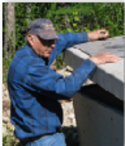
Jarecki installing the vault toilet at Ryan Field.
