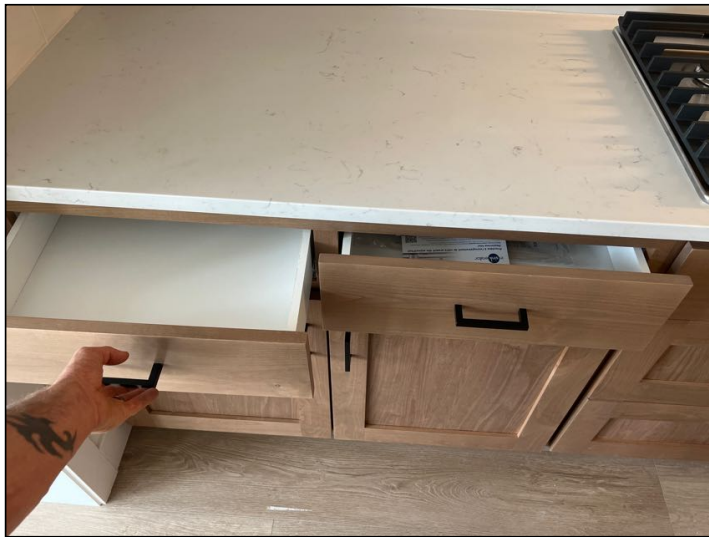
Cabinet drawers appear to be off track and need adjustment- left of cook top and bottom right of sink.
