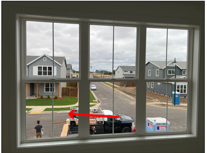
Left side single hung window at upstairs left front bedroom is tight in frame. Recommend adjustment.
