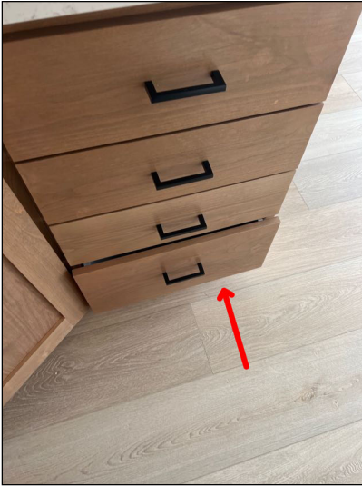
Cabinet drawers appear to be off track and need adjustment- left of cook top and bottom right of sink.
