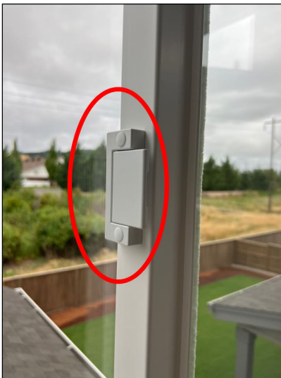
Right side master bedroom sliding window does not latch properly. Recommend adjustment/repair.
