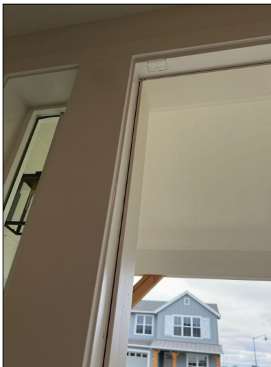
Missing weatherstripping noted at front door. Recommend installation.
