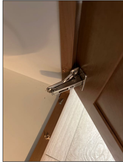
Tighten hinges under sink.
