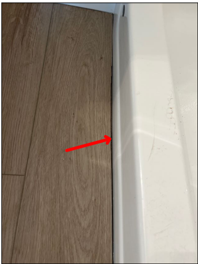
Recommend caulking where the tub or shower meets the floor.
