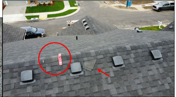
Missing/Damaged shingles at Ridge. Recommend repair by a licensed roofing contractor.
