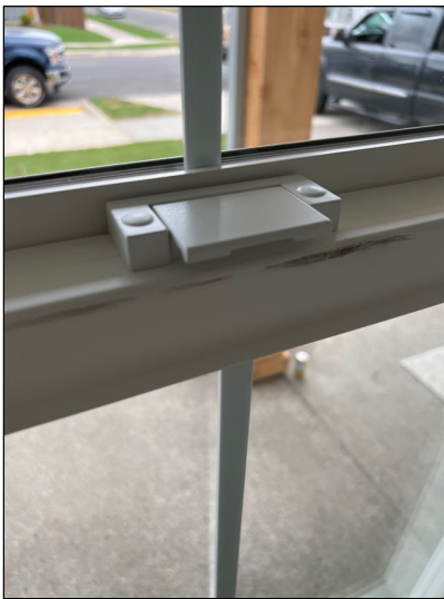
Right side single hung window at main floor right front bedroom does not latch properly. Recommend adjustment/repair.
