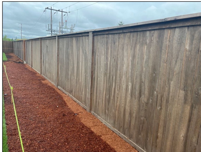
Recommend one inch between soil and fence to prevent decay.
