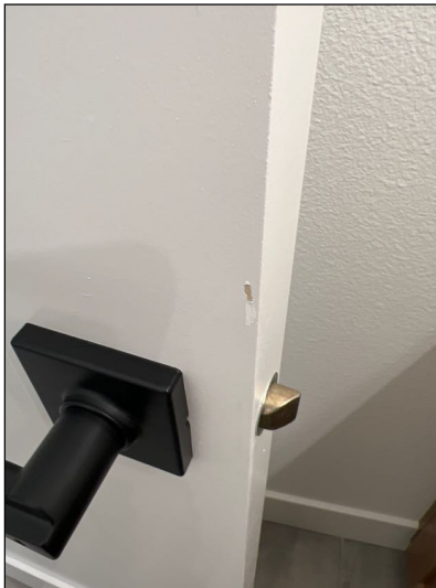
Minor cosmetic damage observed at upstairs hallway bathroom door. Touchup paint is needed.
