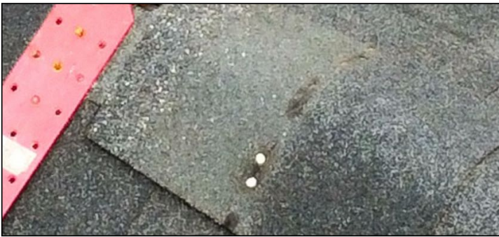
Missing/Damaged shingles at Ridge. Recommend repair by a licensed roofing contractor.
