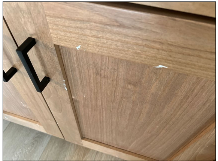
Minor cosmetic damage observed at some cabinets. Recommend repair.
