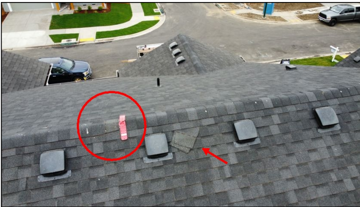
Missing/Damaged shingles at Ridge. Recommend repair by a licensed roofing contractor.
