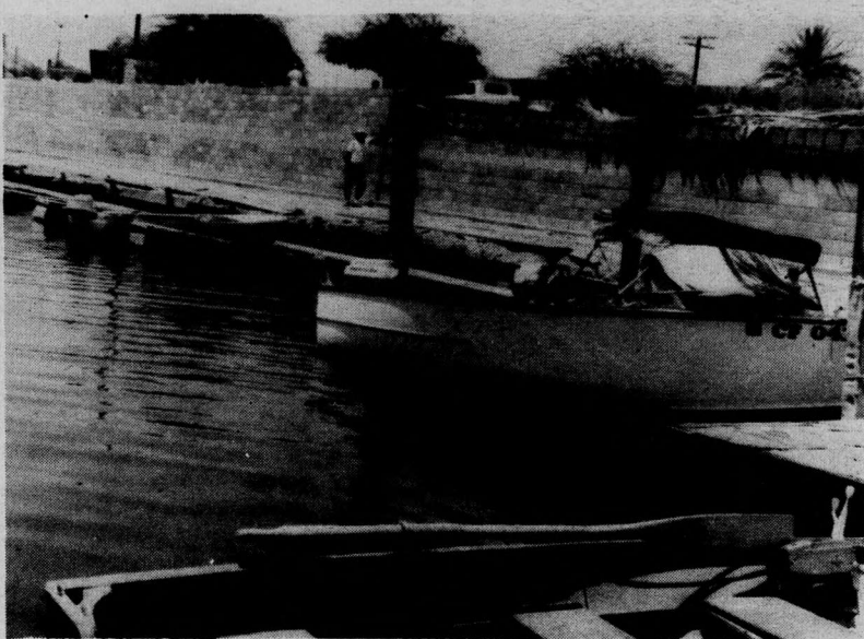
NEW CONSTRUCTION- An 160 ft. wall, 10 ft. high, is now under construction at the Desert Shores Marina, which was the first boat landing at Desert Shores. Here there is a charter boat for fishing. There are gas pumps and a pre mix pump has just been added. There are slips, bait and tackle. A wide drive is planned for the convenience of those loading and unloading at private docks and will run along the base of the new wall.
