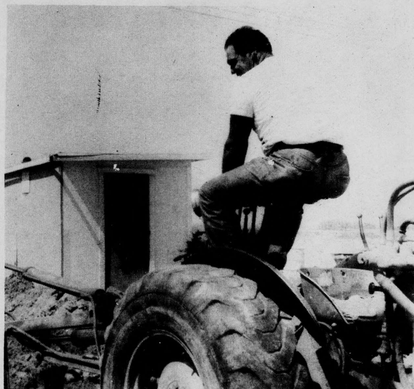
ANOTHER INSTALLATION- Here Larry Whealy, of Salton Sea Beach is preparing for the setting of a septic tank on Brawley Avenue. You may call Whealy for tractor work and septic tank installation by dialing EX 5-2277.
