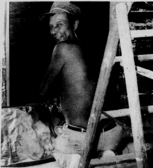
AN ADDITION AT MIKE'S- Chuck Tubbs, of Mike's Tackle Box, insulating the room which will be an extension of the popular beer bar at Mike's Tackle Box, Desert Shores.
